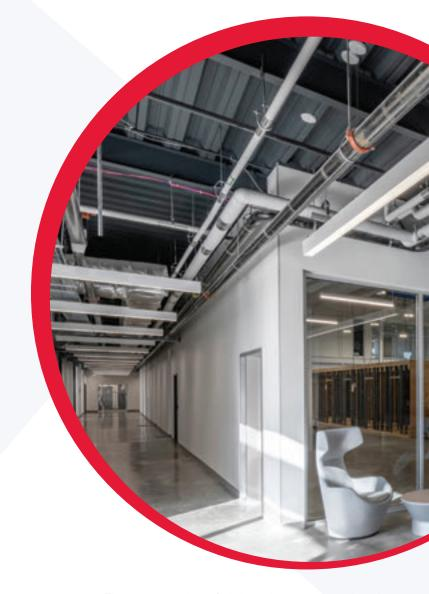
The presentation of visible elements mandated more installation aesthetics than conventional commercial buildings that typically recess everything behind walls and ceilings, according to Newham. Ductwork mastic, for example, tightly seals ductwork connections, but in this case it had to look perfect.
