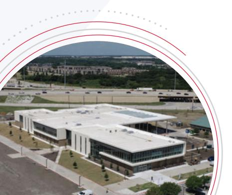
Keeping the AHUs, DOAS and other equipment indoors also complied with the City of Coppell's building code that restricts rooftop clutter. The CSB's roof is very visible from adjacent elevated "gateway to the city" Highway 121 and nearby DFW International Airport air traffic.
